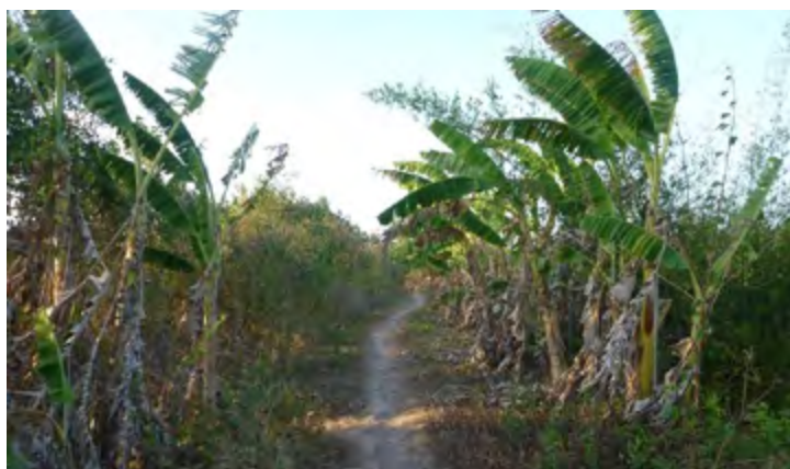
Fig. 8b. Earthen sea-dyke along the West Sea coast of the Mekong Delta in Kien Giang province. The dyke crown is cultivated with banana trees and other crops since berm and crown are less harmed by saline water intrusion. However, certain crop cultivation with deep root systems and trees might lessen the stability of the dyke surface and should be avoided.
