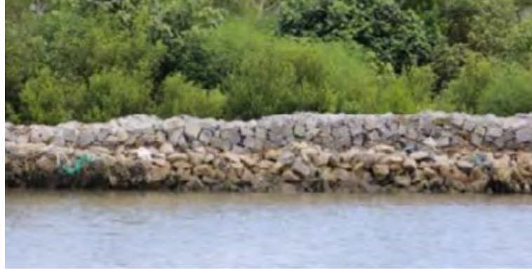
Fig. 21. Gabion revetment. Source: Phan Thanh Tinh
