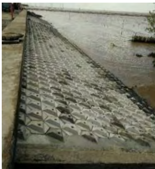
Fig. 27. Concrete slab armoured sea-dyke. Source: Phan Thanh Tinh
