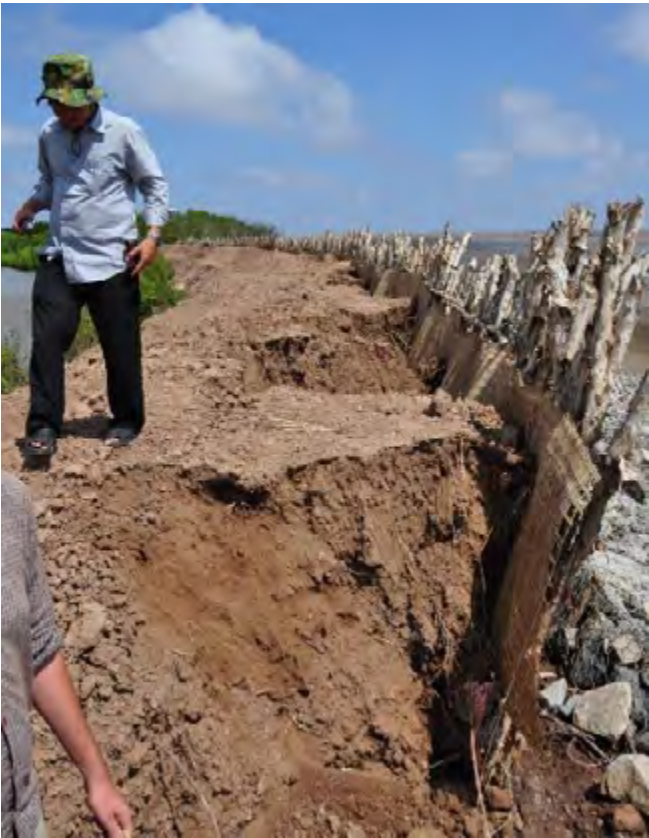
Fig. 40. Typical sea-dyke failure along the East Sea coast of the Mekong Delta. Once an earth dyke with very steep profile and a lack of toe protection is exposed to even moderate wave surge, the dyke is undermined and collapsing towards the seafront. Longer periods of storm surge with high water setups and wave overtopping would destroy the sea-dyke in a very short period. Source: Frank Thorenz
