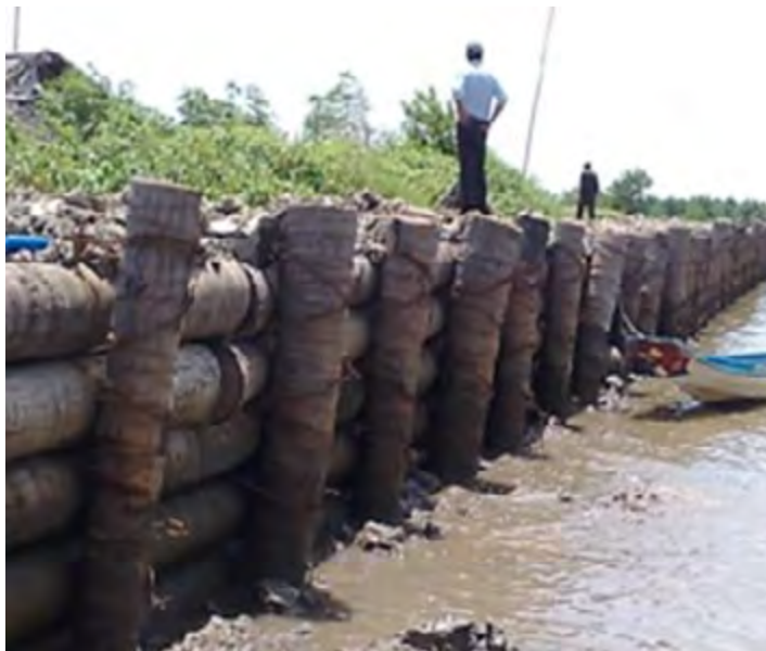
Fig. 22. Coconut lumber seawall. Source: Phan Thanh Tinh
