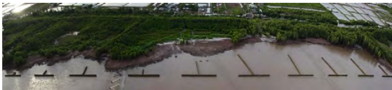
Fig. 47. Restoration of eroded floodplains using bamboo T-fences in Bac Lieu Province (Mekong Delta, Viet Nam). The long-shore elements close the eroded gap in the mangrove forest by connecting the remaining headlands. Photo Cong Ly and G.E. Wind 2013. Source: Cong Ly và G.E. Wind 2013
