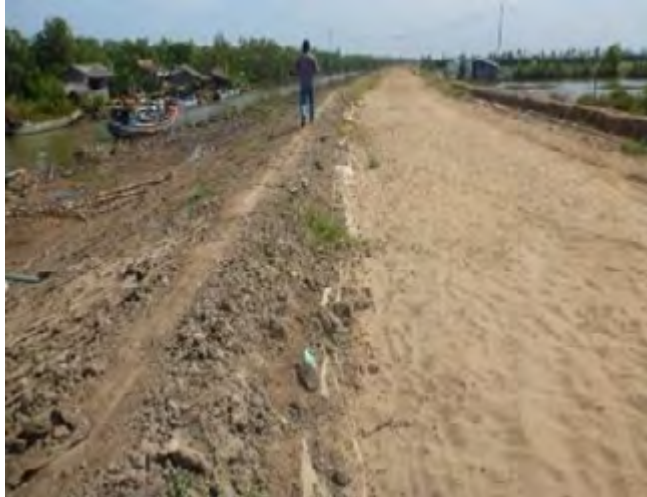
Fig. 32. Strengthened earth dyke. Source: Stefan Groenewold
