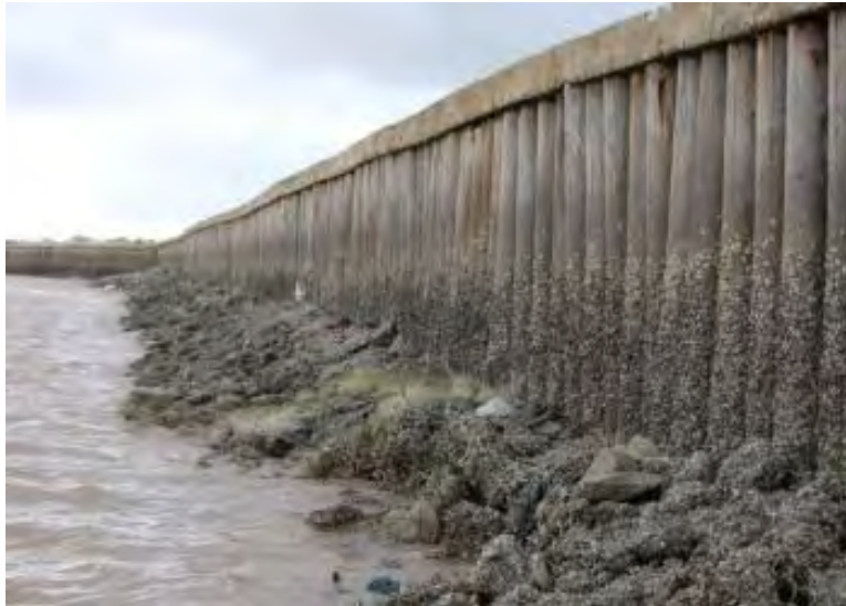
Fig. 24. Concrete pillar seawall.
