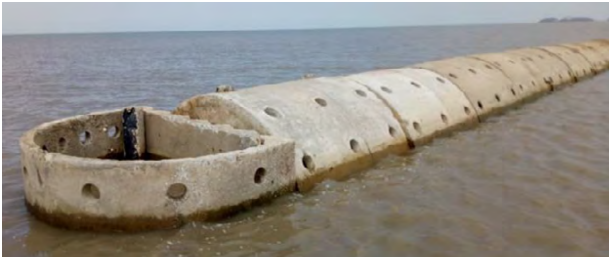
Fig. 12. Detached “hollow dyke” breakwater. Source: Frank Thorenz
