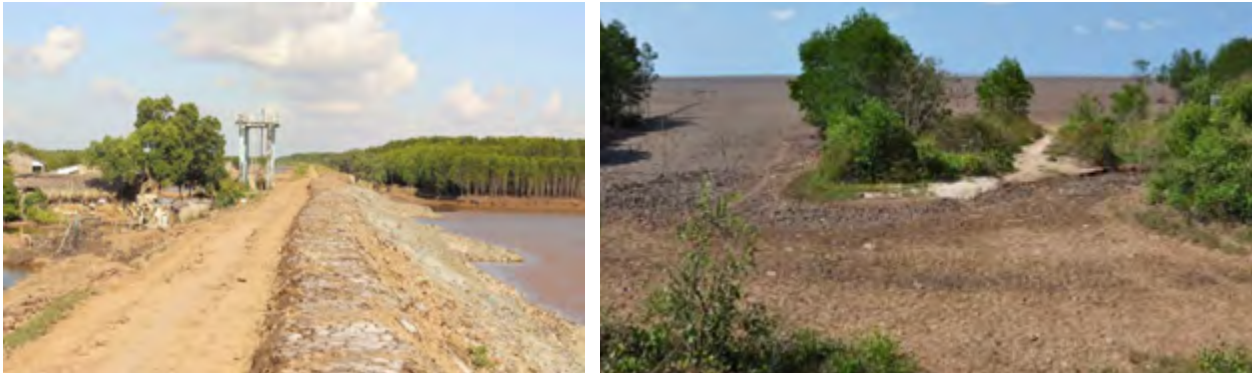
Fig. 38. Typical sea-dyke profile with riprap revetment and foreland in the Mekong Delta in Vietnam (East Sea). The conservation of dyke-foreland is of high importance for the resilience of the dyke. Source: Frank Thorenz
