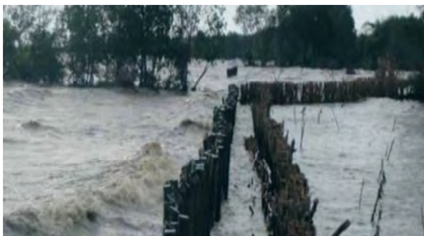
Fig. 16. Sediment trapping double-fence. Source: Stefan Groenewold
