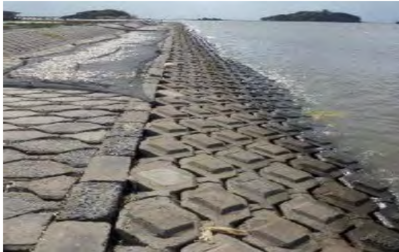
Fig. 29. Concrete slab armouring. Source: Stefan Groenewold
