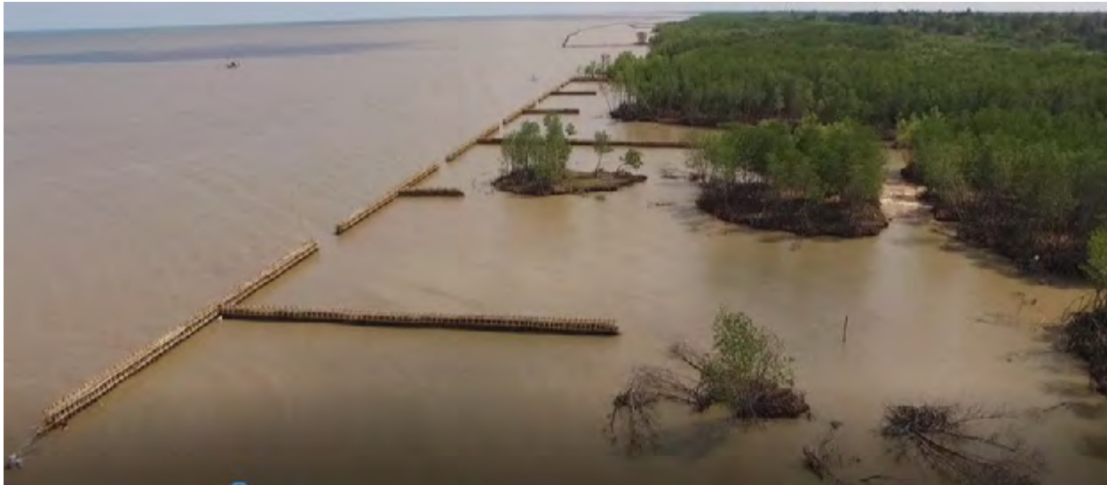
Fig. 65. Ca Mau, T-fences in the West Sea. Source: Ca Mau Department of Agriculture and Rural Development
