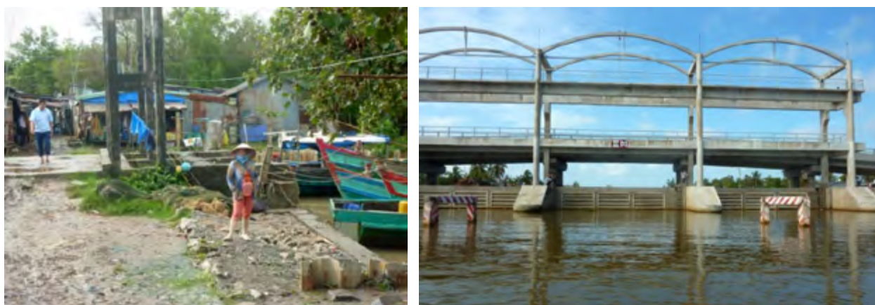
Fig. 34. Sluice gates. Source: Stefan Groenewold
