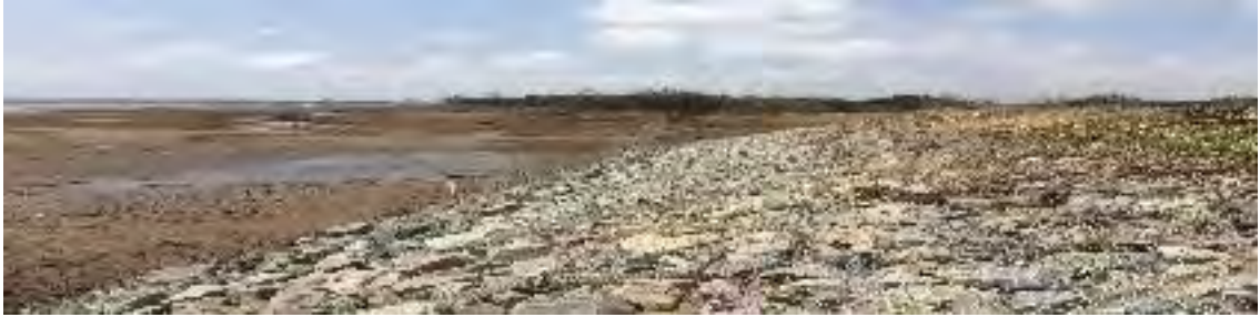
Fig. 25. Gabion revetment of sea-dyke. Source: Holger Schuettrumpf & Peter Froehle
