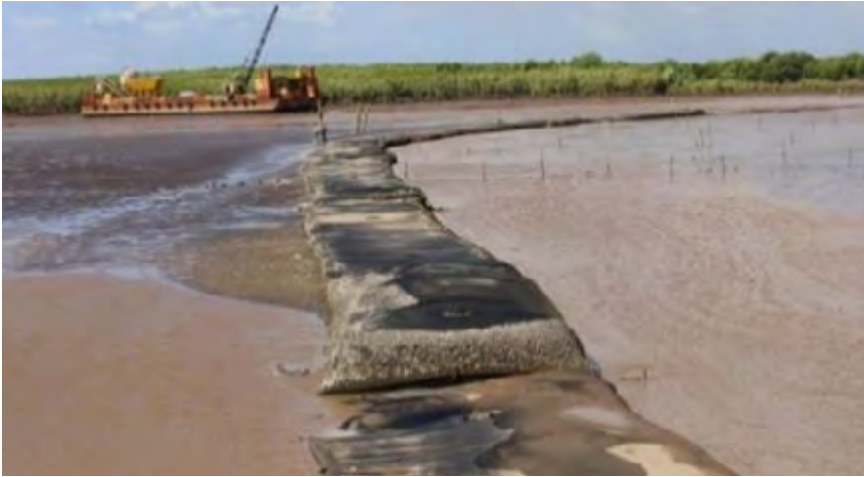
Fig. 14. Detached geotextile breakwater. Source: Frank Thorenz
