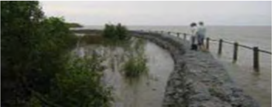
Fig. 20. Gabion breakwater. Source: Phan Thanh Tinh
