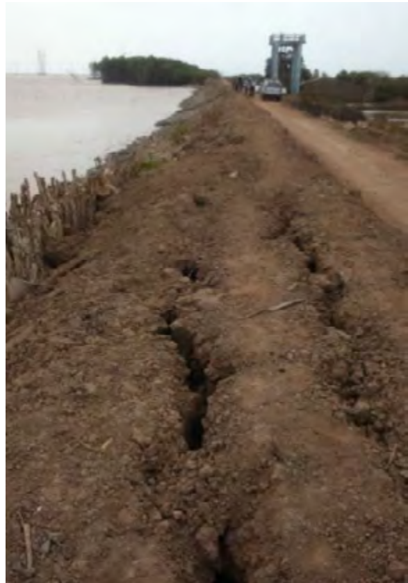
Fig. 40. Typical sea-dyke failure along the East Sea coast of the Mekong Delta. Once an earth dyke with very steep profile and a lack of toe protection is exposed to even moderate wave surge, the dyke is undermined and collapsing towards the seafront. Longer periods of storm surge with high water setups and wave overtopping would destroy the sea-dyke in a very short period. Source: Frank Thorenz
