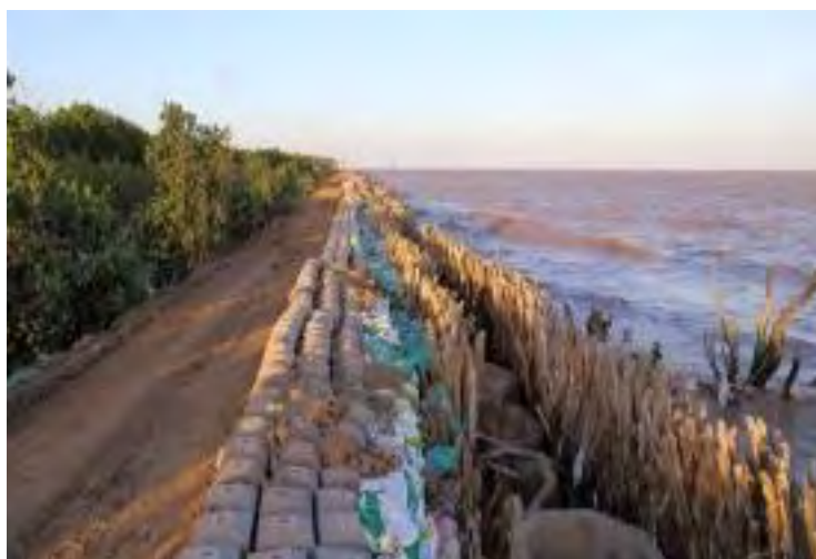
Fig. 26. Mixed emergency sea-dyke revetment. Source: Holger Schuettrumpf & Peter Froehle
