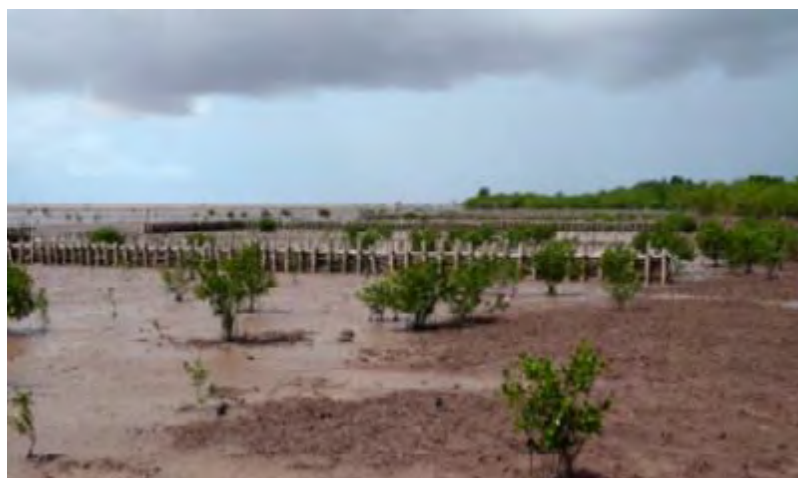
Fig. 15. Mixed breakwater and groyne fields.
